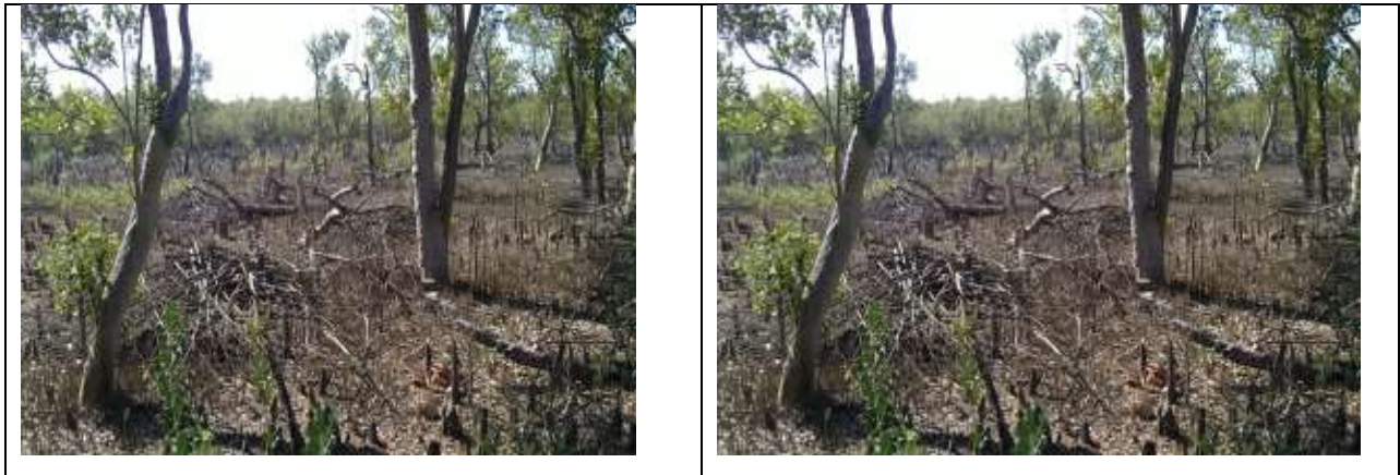
Tree cutting and land cleaning
