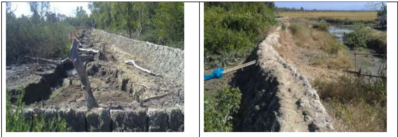
Embankment or dyke construction
